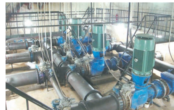
太原市汾河景区绿化美化工程加压泵 Taiyuan Irrigation Project (ISG125-300 250m³/h @ 30m @ 30kw)
