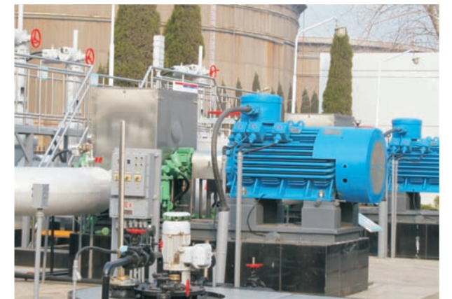
中石化管道储运分公司南京输油处石埭桥泵站 Sinopec Pipeline company Nanjing oil transportation Shihuqiao Pump station TSY250-200-520(Q=750m 3 /h,H=50m P=160kw)
