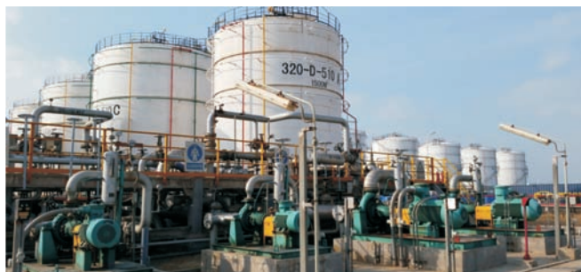
青岛丽星仓储化工有限公司TCE(OH 2 )装船泵 Qingdao Li Xing Storage Chemical Co., Ltd. TCE(OH 2 ) Shipment Pump
