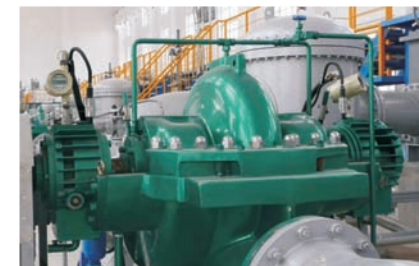
大连国家石油储备油库汽油泵 Dalian National Oil Stock Project (TSY400–300–700 1500m³/h @ 100m @ 560kw)
