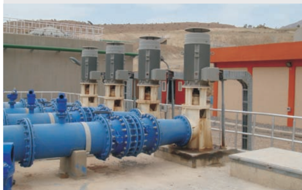
山西万家寨引黄工程排水泵 Shanxi Wanjiashai Yellow River Project (300TTV 210-11x9 210m³/h@95m@ 90kw)
