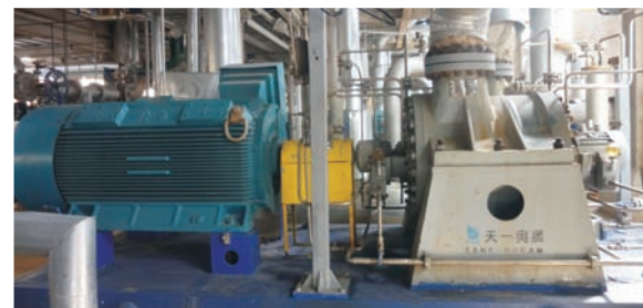
腾龙芳烃脱丁烷塔回流泵 Dragon Aromatics (Zhangzhou) Co. Ltd. Debutanizer Reflux Pump TSJH250-700 ( Q=800m 3 /h,H=147m,P=355KW )
