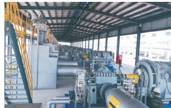
董潍管线 Dongwei Line (TSY400–350–435 2300m³/h @ 210m @ 1600KW)
